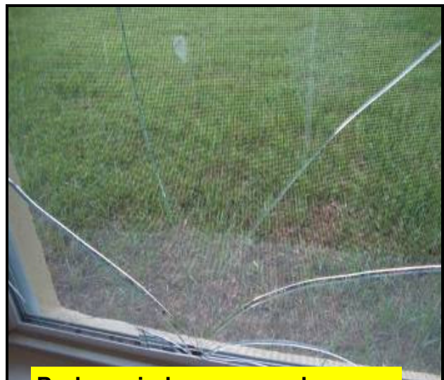
Broken window pane on lower sash - garage window (page 3, J).
