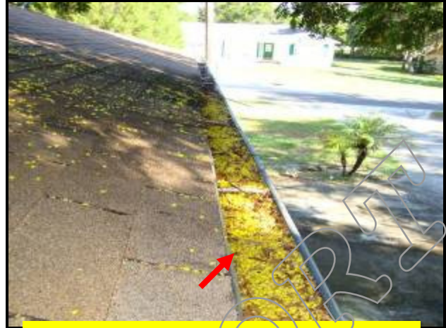
Gutters full and causing anchors to pull away from home (page 2, F.)
