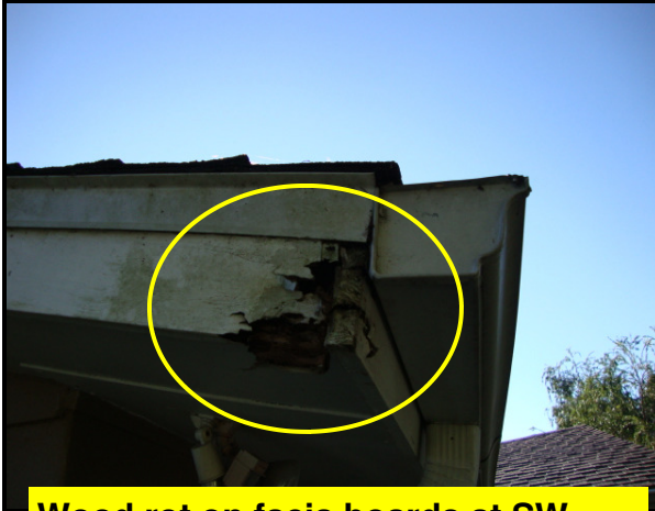
Wood rot on fascia boards at SW corner of home (page 2, E.)
