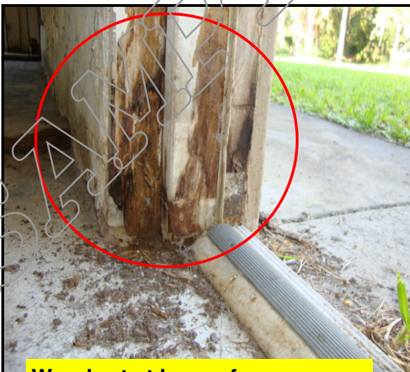
Wood rot at base of garage service door jamb (page 3, G).
